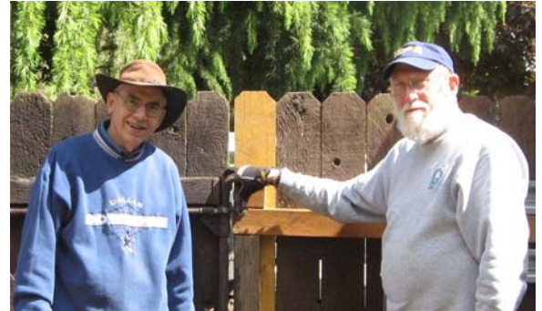
Dave and Bill with their finished gate at Done in a Day
